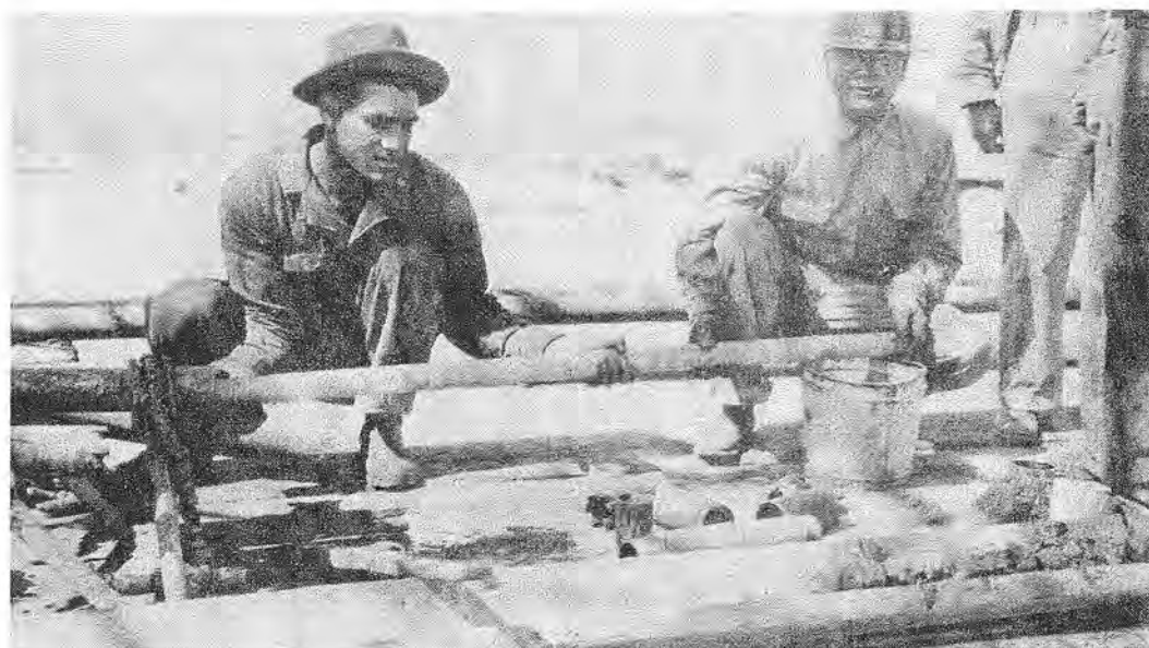
Figure 8. - Removing salt core from core barrel.
